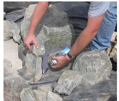
Use expanding foam to fill in voids between rocks
