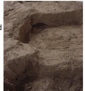
Sculpt and compact dirt in stream area before installing liner
