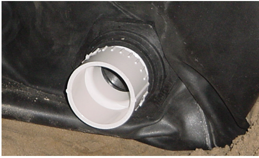
Bulkhead is through liner, washer/nut are tightened and PVC adapter is installed.
