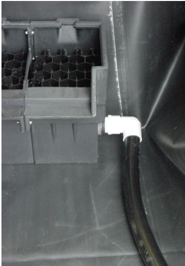
Bulkhead is through liner, washer/nut are tightened and PVC adapter is installed.
