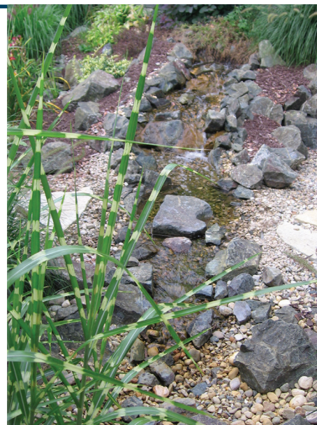
Once large rocks are placed and any foam work is done, sprinkle 1"-2" stone over stream rocks to fill in voids and cracks.
